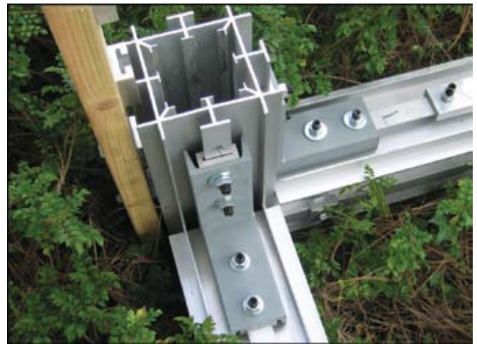
The unique profile of the Modular Housing System aluminum framing extrusions provides channels which enclose the edges of SIP or other panels and allow connections with other members anywhere along their length.
